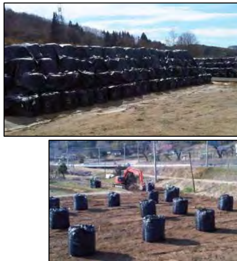
Figure 13: 1m 3 bags of soil in the field, and temporary storage.
