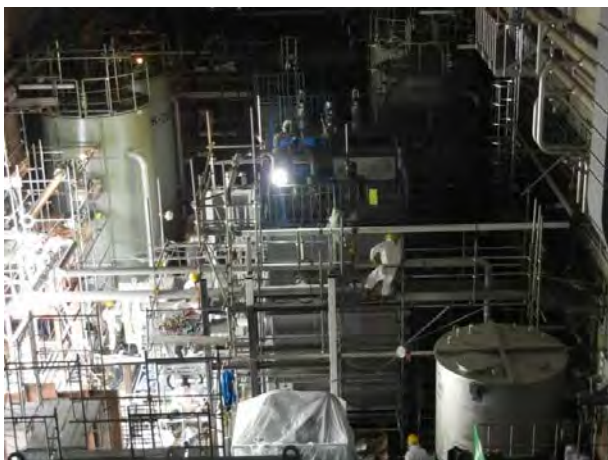
Figure 2: AREVA water processing unit.
